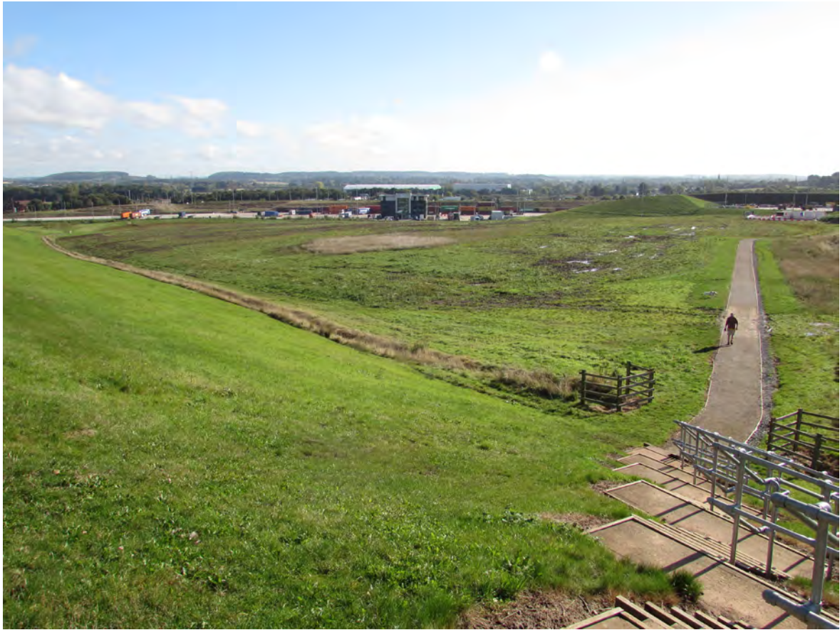
Plate 7: View of the Western Part of the EMG1 Works Looking Northeast
