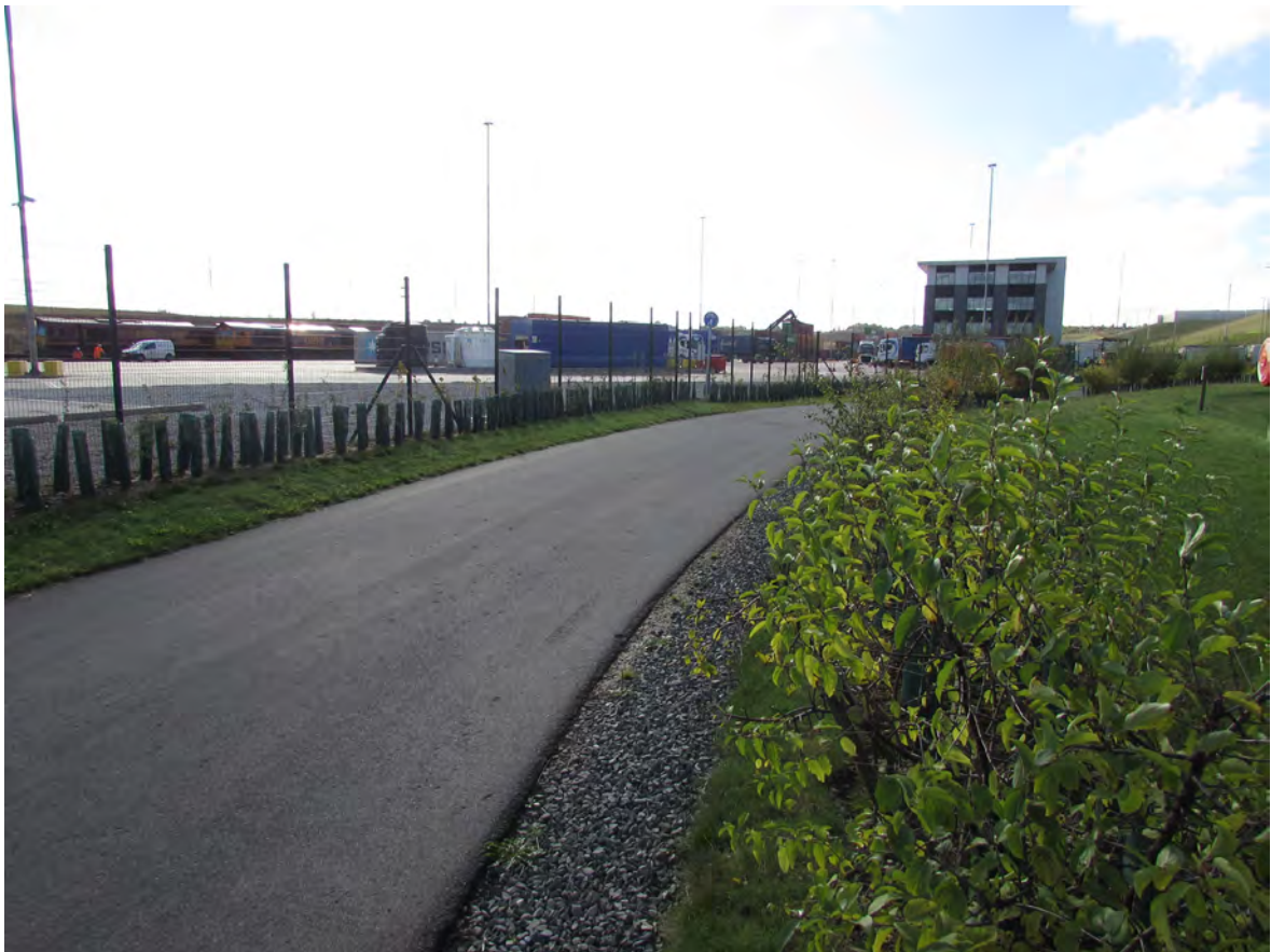
Plate 8: View of the Eastern Part of the EMG1 Works Looking Southeast
